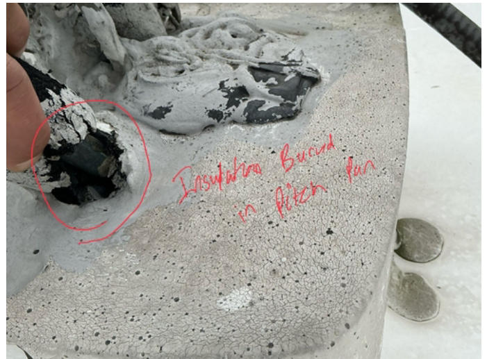
AC Chase with insulation buried in Pitch Pan. When line insulation above pitch pan deteriorates, water follows copper AC line through pitch pocket into interior. Proposal includes checking and resealing all AC lines.
