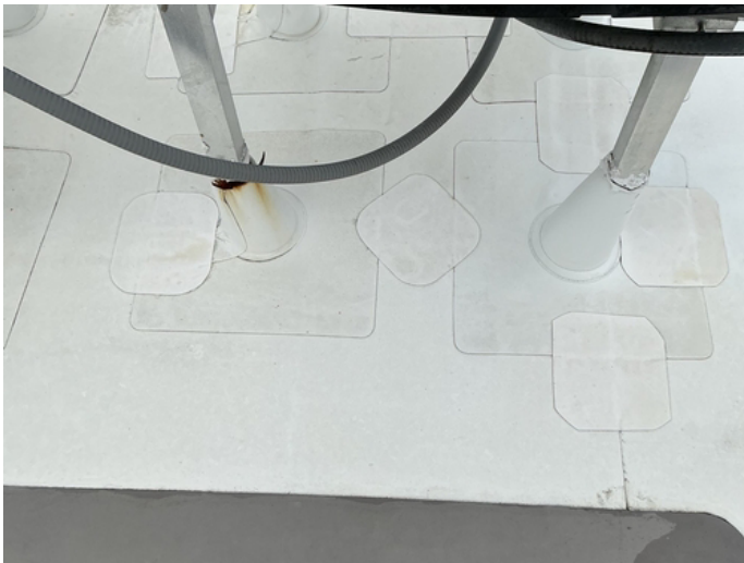
Rusted boot clamp. This proposal includes resealing all AC Stand penetrations.
