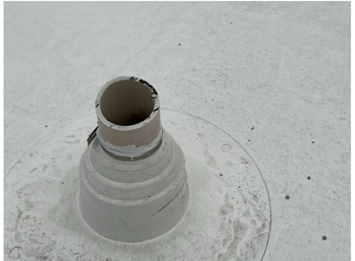
Some penetrations have cracked sealant. This proposal includes resealing all penetrations.
