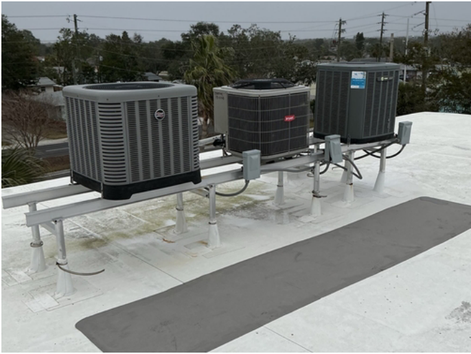
When boots were resealed, contractor did not cut off excess clamps. This proposal includes removing excess clamps and resealing all AC pipe boots.
