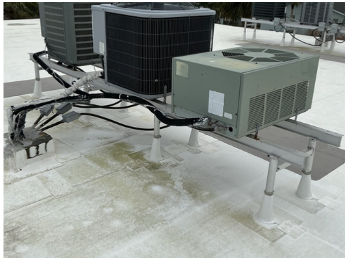
Some AC stands are still sealed. This proposal includes cleaning up old sealant and resealing all AC stands for longevity.
