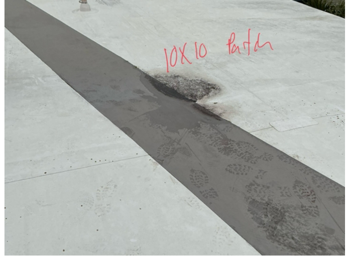
Ponding - Cut membrane, excavate ISO, new ISO with appropriate slope to gutter, new membrane.
