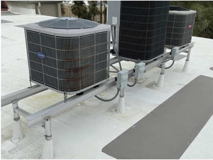
Missing Pipe Clamp - This proposal includes cleaning up old sealant and resealing all AC stands for longevity.
